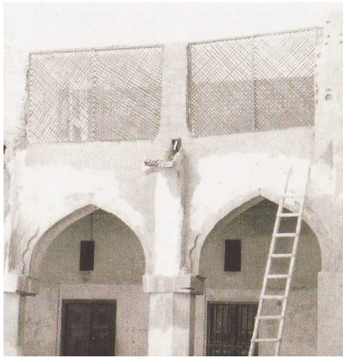
Figure 85 Al-Khalid house, wooden lattice parapet wall, 1960. Source: Lautrette, 2006.
